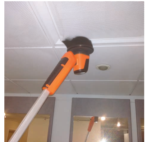
Ceilings & Ventilation Grilles
